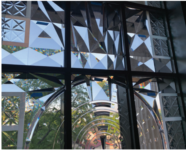
The highest parts of the windows are the “crescendo” of the space, incorporating almost exclusively prismatic glass in a complex arrangement that throws refracted light through the main foyer. Each prism was individually designed, molded, and polished, then laminated to a quarter-inch-thick pane of tempered glass. The top-middle rectangle, the most complex, includes twenty separate prisms.
